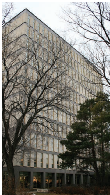
The Arts Tower is one of the core campus buildings in need of major renewal.
