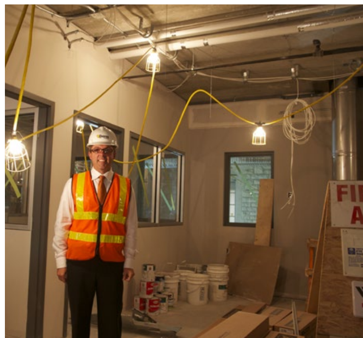
Derrin Raffey amid the construction of the STM addition.
