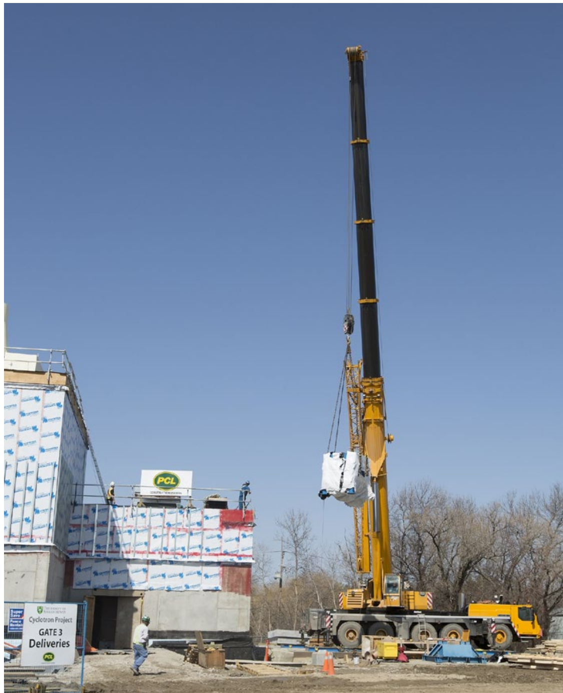
The cyclotron is lowered into its concrete vault.
