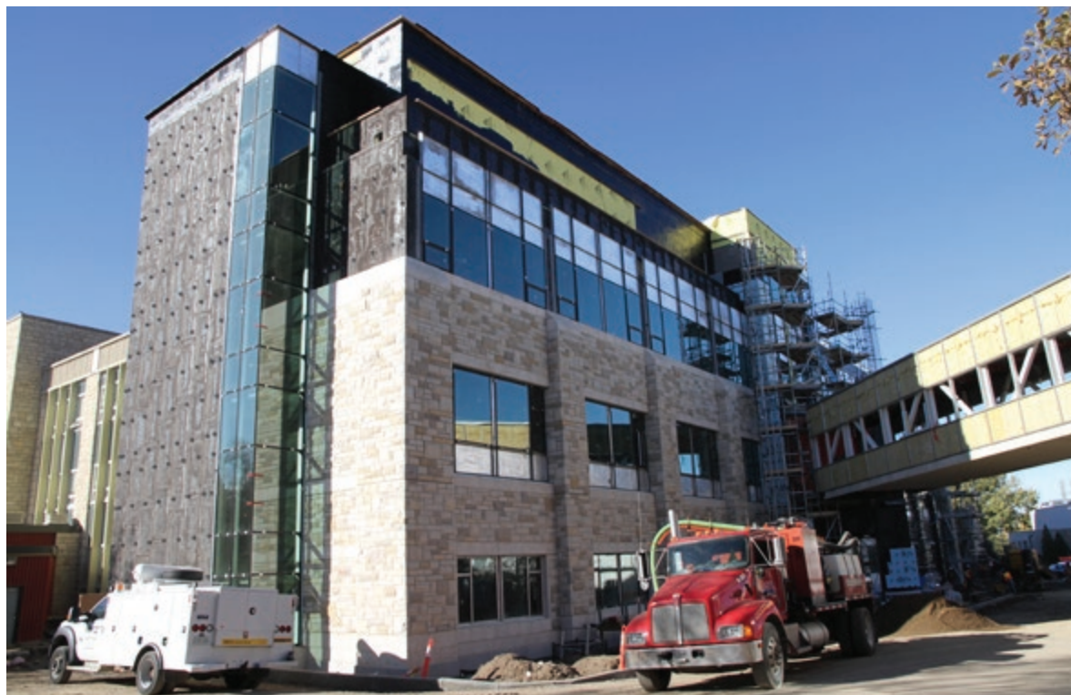
Construction is continuing on the new state-of-the-art Collaborative Science Research Building.
